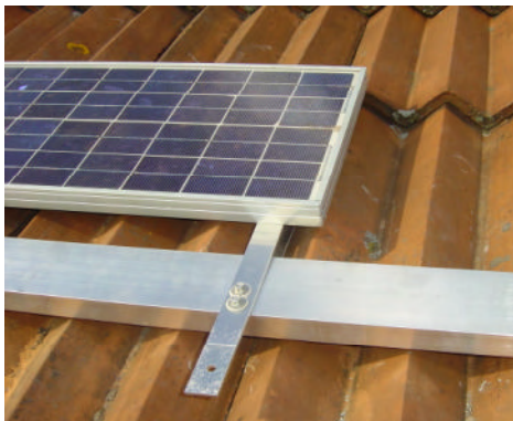
A5 Figure 6: PV module mounting
