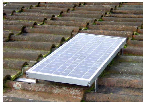
A5 Figure 3: Completed Installation with frame
