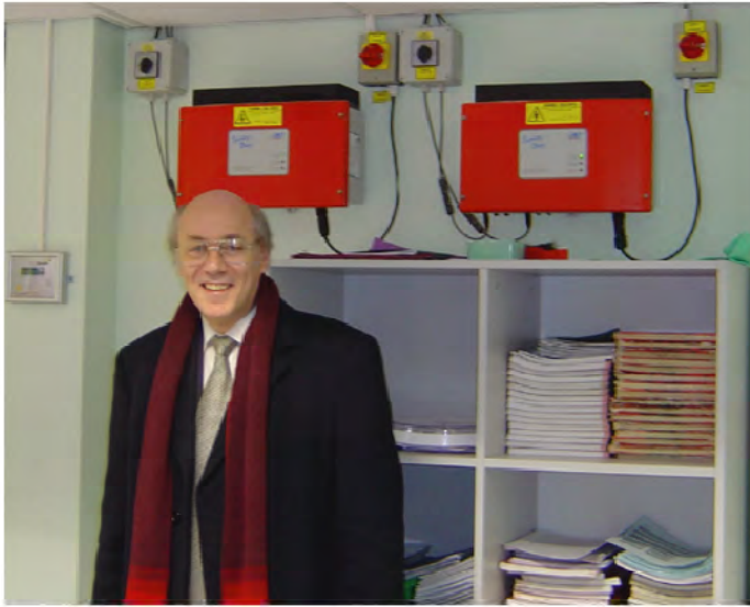
Dr Tim Hooker by inverters and meter for photovoltaic system
