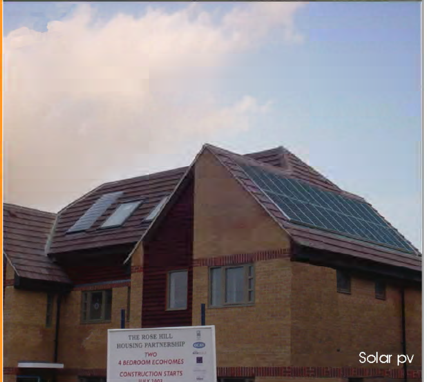
Installed by accredited agent, South West Trace Heating
